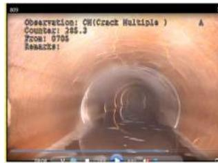
Cracking – Pipe ID 12551
